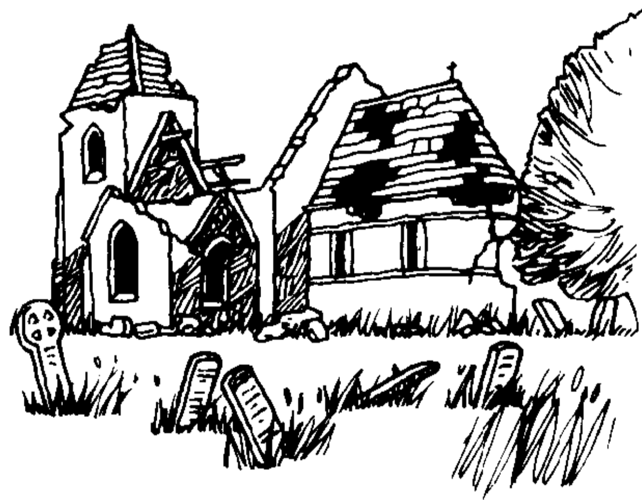
The old church is falling down.
